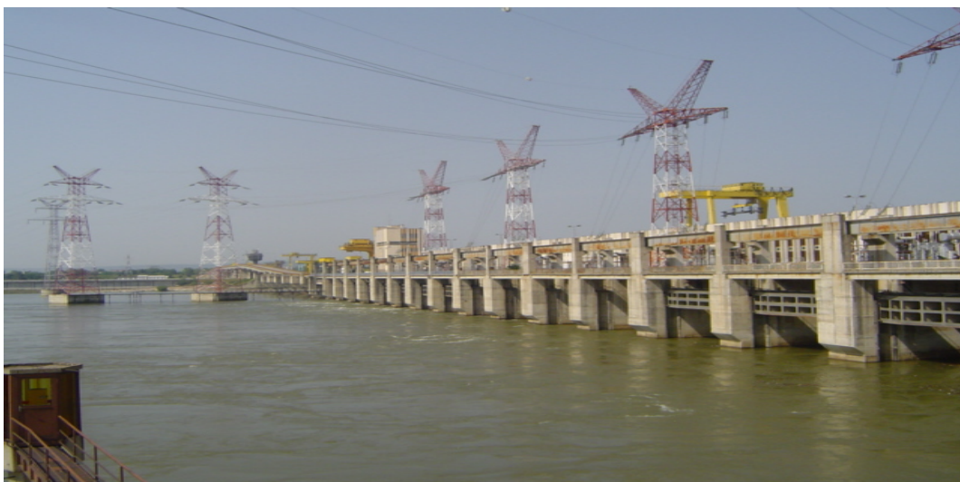
Fig. 2 The dam of « Iron gates » is with 2100 MW the most powerful hydro power plant of Europe and produce 12% of the Rumanian electricity power. The dam was built between 1965 and 1971.
